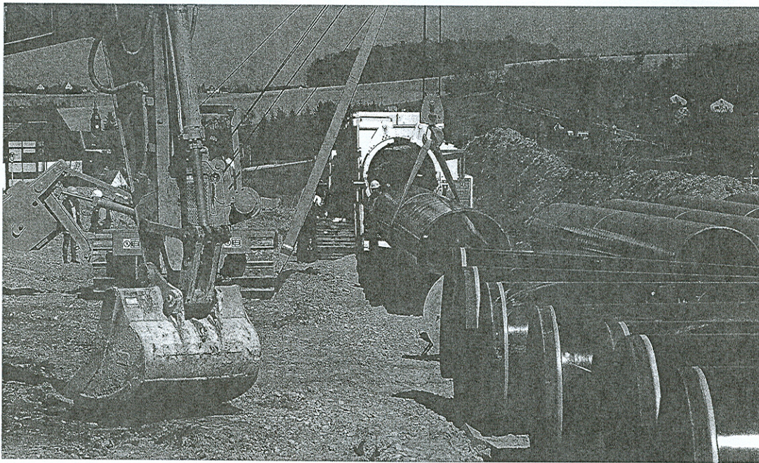
Liebherr machines working on a gas pipeline in Saxony, Germany.
